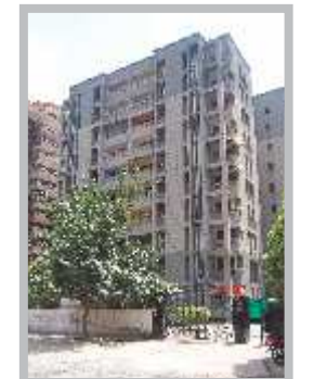
Anuradha Apartment, Vaishali
